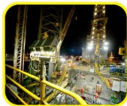
Petrol Process Factory
